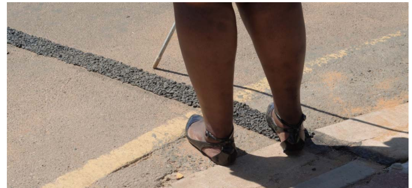
Figure 10: Recommended rumble strip that was installed for testing in Tshwane on 17 th Nov 2016, served as a very useful assistive feature for people who are blind to enable them to cross the road successfully
