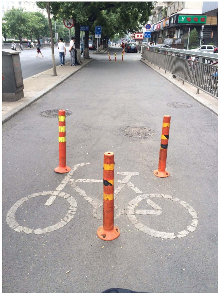
Figure 14: Bollards at Cycle Path to avoid abuse by motorised vehicles. Source: http://www.juca.org.za/?paged=8
