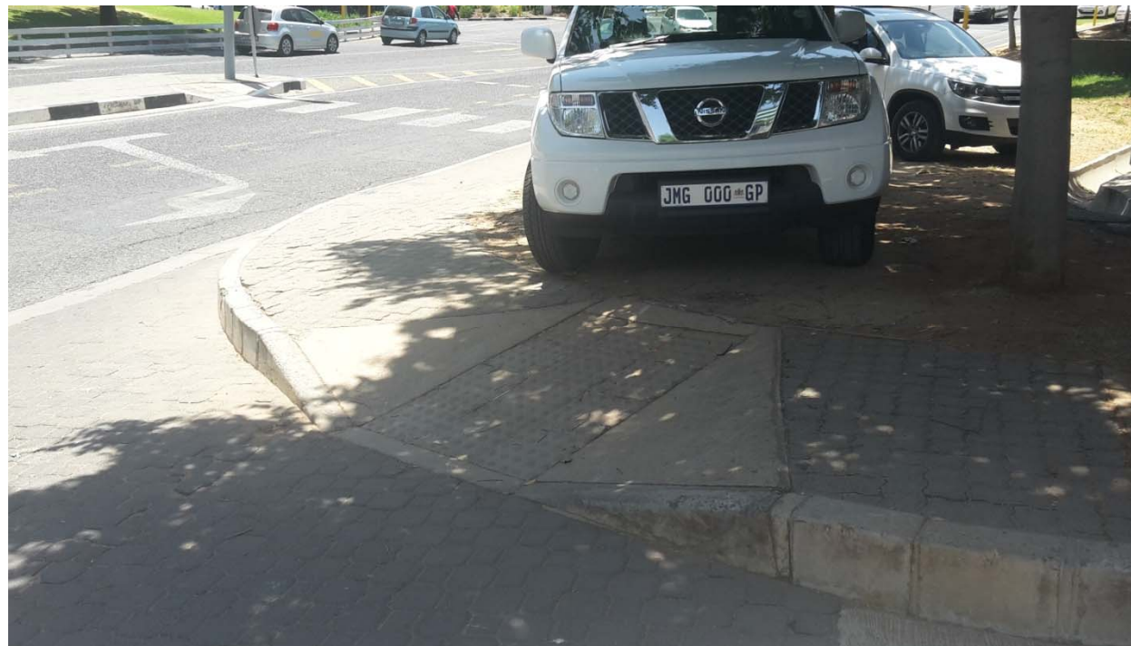
Figure 8: The misuse of kerb cut areas by vehicle drivers is common at both signalised and un-signalised intersections. Bollards, and the installation thereof, are recommended but not listed as a technical requirement for NMT1 and, therefore, remain the prerogative of the designers/engineers or Municipality. If bollards are to be installed it is recommended that they be installed according to the drawings in other parts of this NTR1 document
